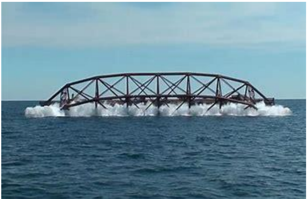
Photo 2-DuPont Bridge Deployment Photo by FWC
